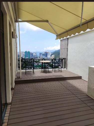
Completed site photo 1.
